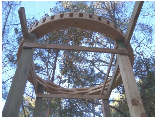
Ceiling ring in place ready for insertion of rafters.
