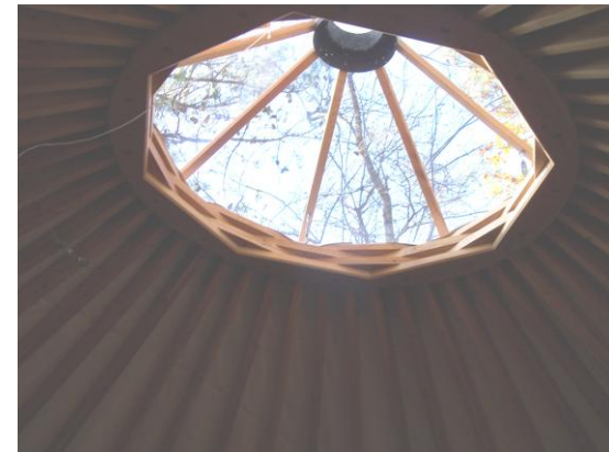
View of skylight and rafters from inside.
