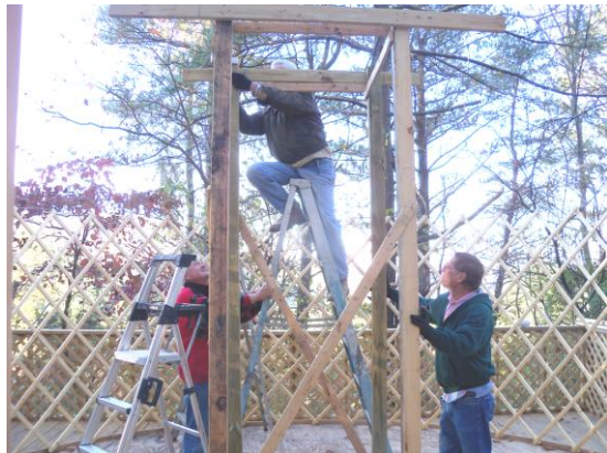
Jim Howling Wolf Allison, Rick Runningbear, and Mike Stonecarvr prepare platform to support center roof ring.
